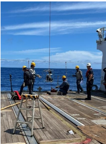
An in-situ pump, brought from MARUM Center for Marine Environmental Sciences, University of Bremen, is deployed from research vessel KAIMEI for particulate organic matter sampling. JAMSTEC ©
